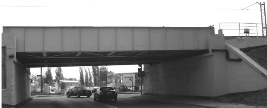
Fig. 4. General view of the railway viaduct
